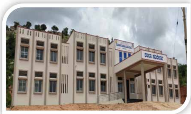
Construction of 3 BHK Housing units
