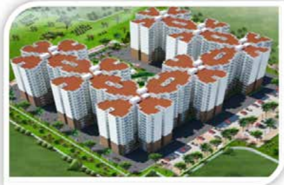
Construction of 1000 bedded Ward Block
