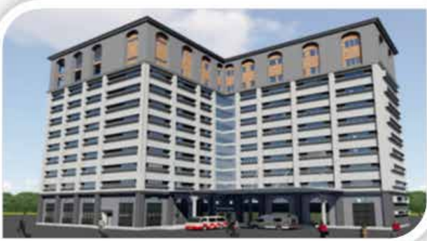
Construction of 3 BHK Housing units
