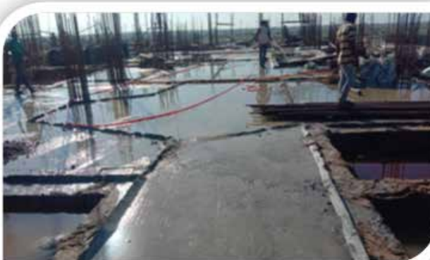
Construction of 3 BHK Housing units
